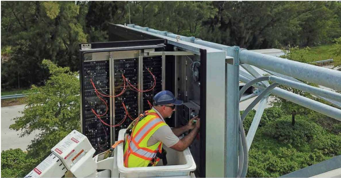
ITS maintenance technician repairing a DMS
