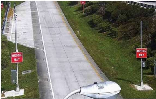
WWDS along southbound I-95 off ramp to NW 95 th Street
