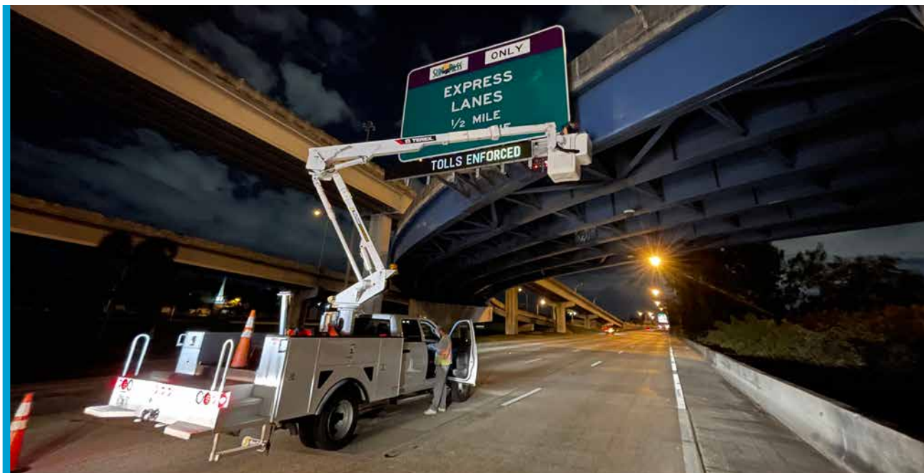
ITS maintenance technician repairing a DMS
