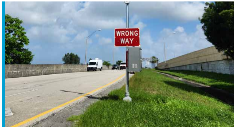
WWDS along southbound SR 826 off-ramp to SW 56 Street
