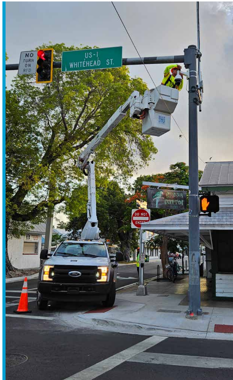
Keys COAST camera installation in Key West
