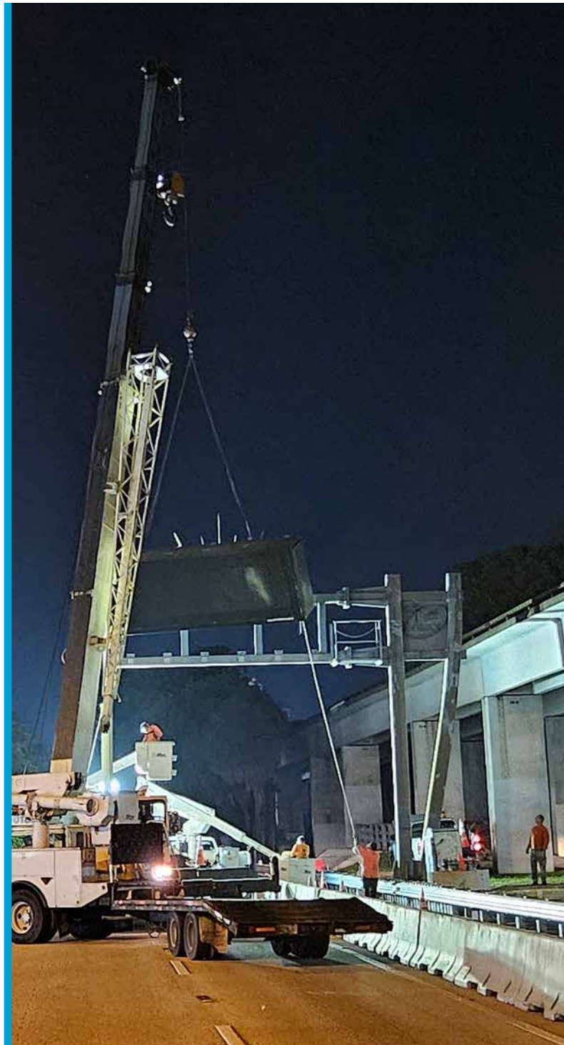
DMS replacement along US 1
