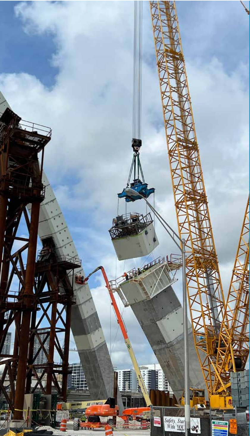
Installing segments for Signature Bridge arches
