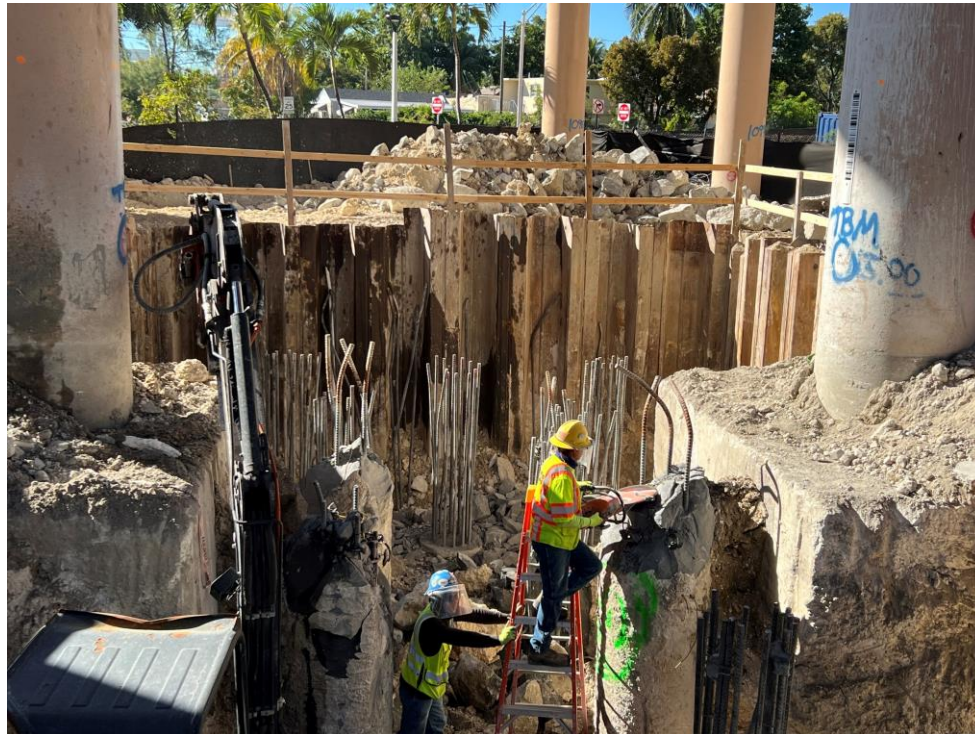
Ongoing foundation and pier cap construction in the Grove Park area
