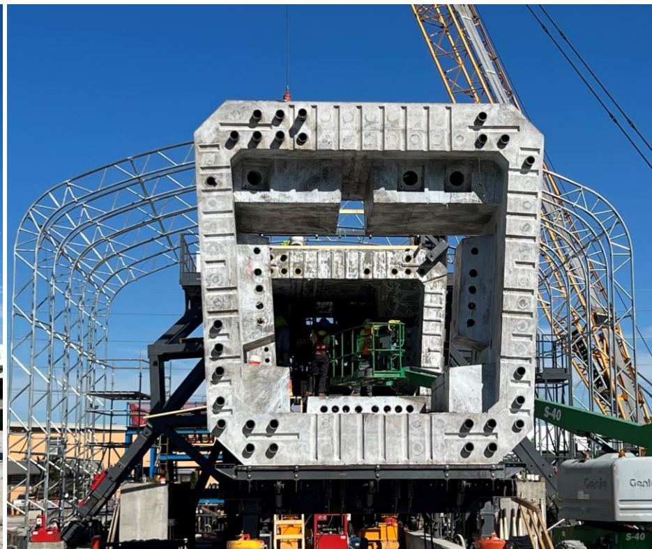
15/345 I-395 Signature Bridge arches cast
