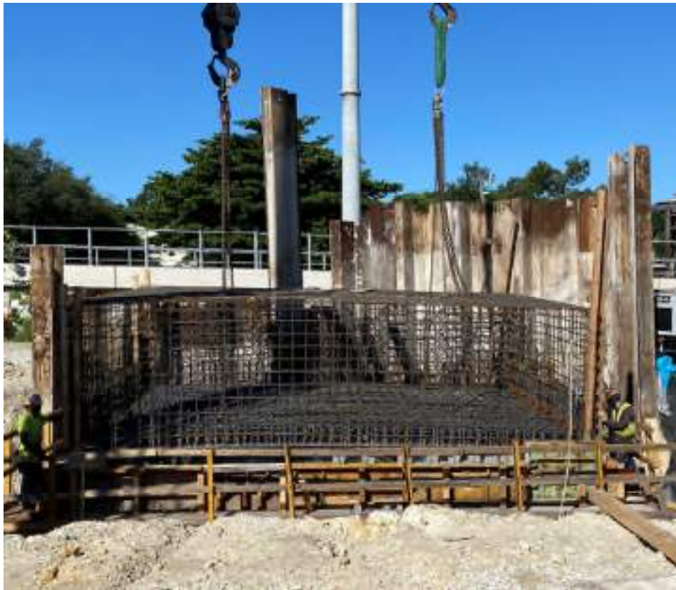
Footer and pier construction along I-395 corridor
