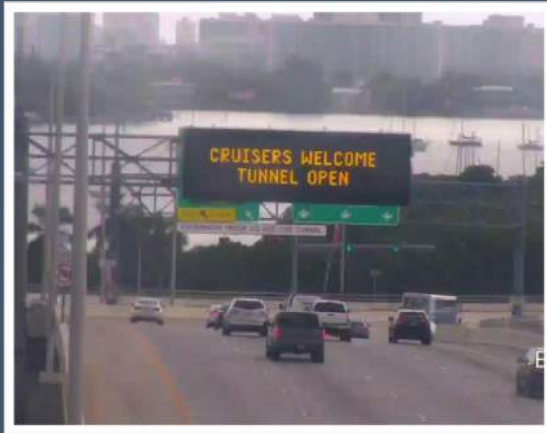
Dynamic Message Sign (DMS) Before Tunnel Entrance
