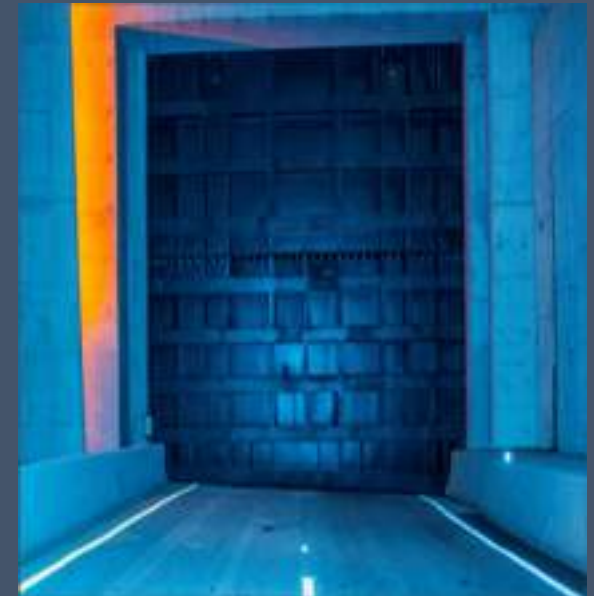
Flood Gate Closed
