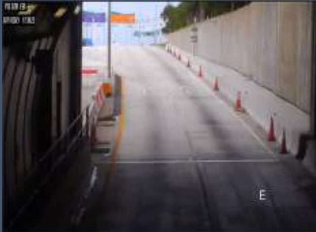
Enters EB Tunnel Exit
