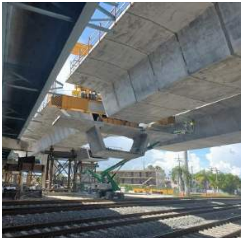
Segment lifter setting segments for new I-395 bridge over FEC/Brightline rail tracks
