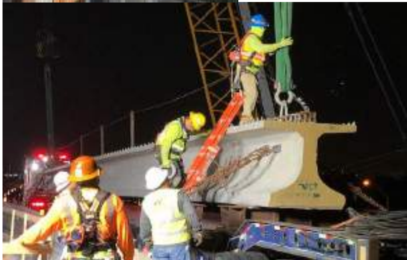
Bridge 108 Reconstruction – Beam Erection
