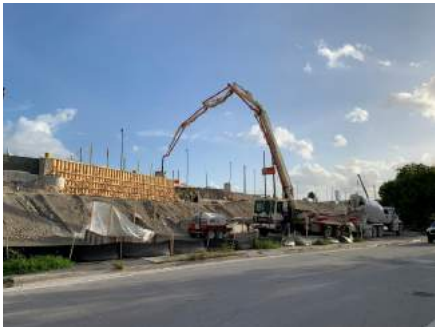
Widening on SR 836 from NW 10 Avenue to I-95
