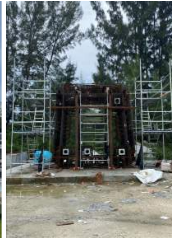
Arch rib reinforcing steel mock-up
