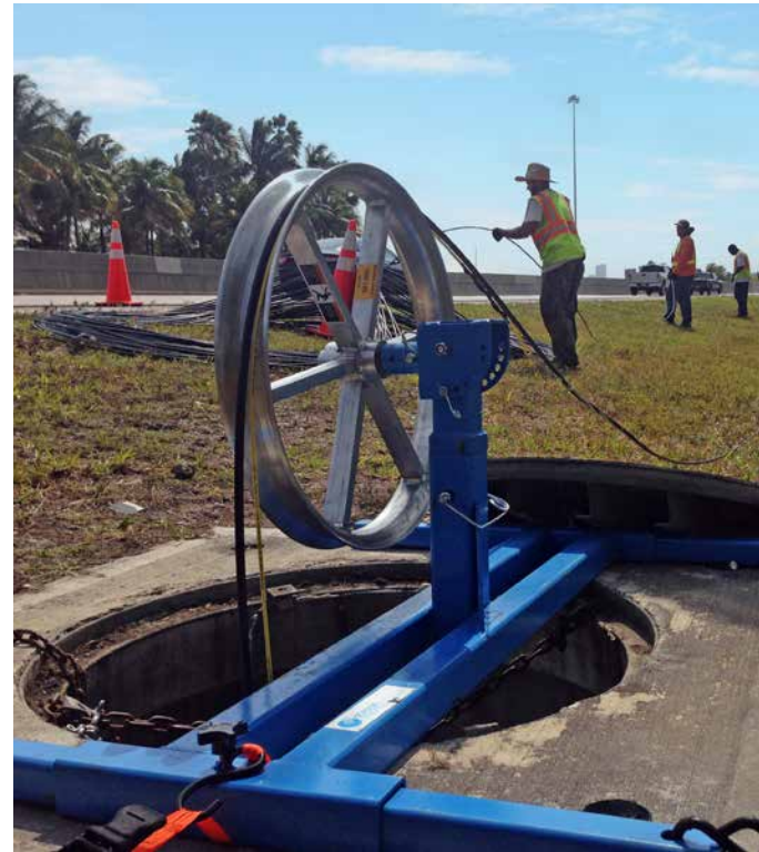
Fiber optic cable installation
