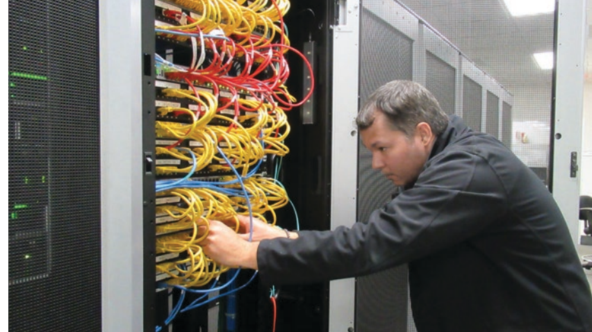
IT TECHNICIAN CHECKING FIBER OPTIC CONNECTIONS
