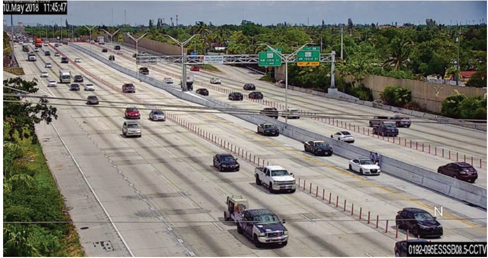
NEW ESS ALONG 95 EXPRESS
