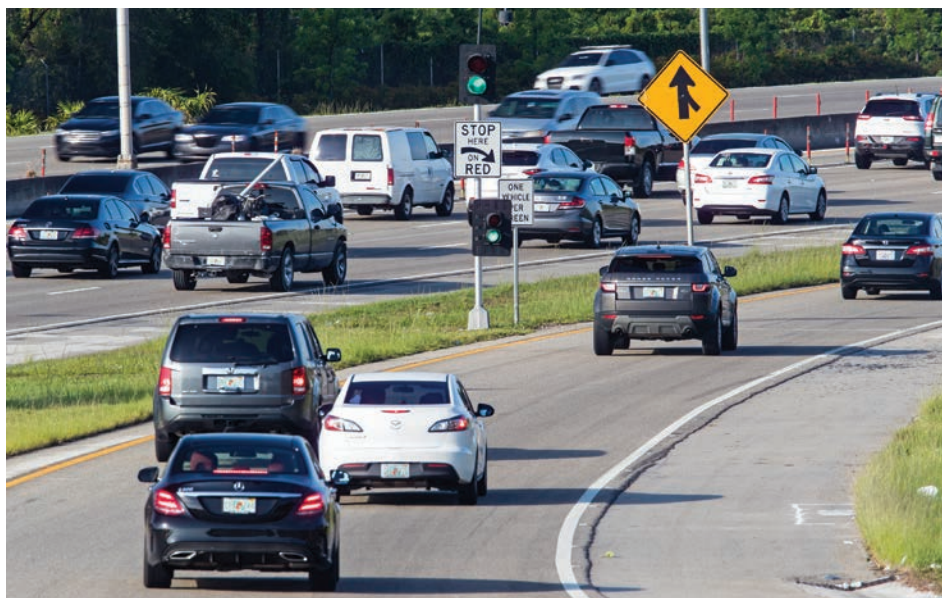
RAMP SIGNAL ALONG I-95
