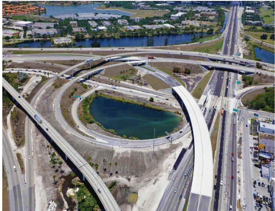
I-75 AND SR-826 INTERCHANGE
