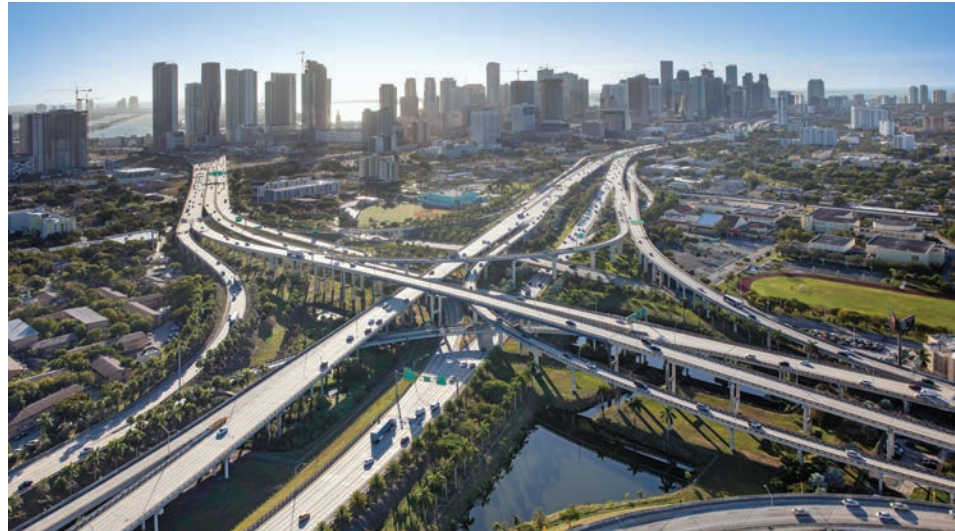
I-95 AND I-395 INTERCHANGE
