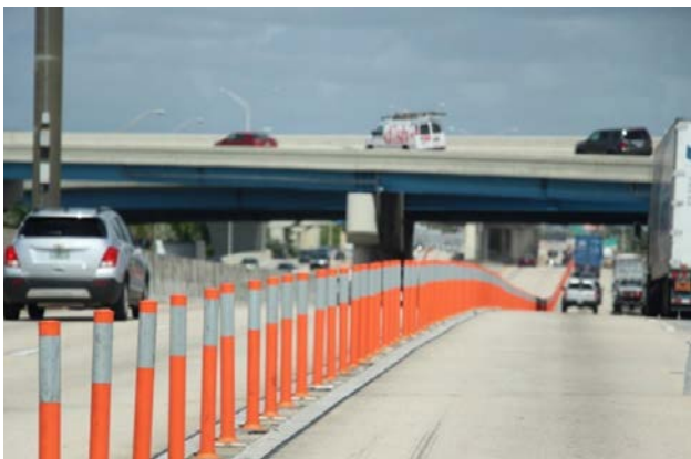
NEW ELMs ALONG 95 EXPRESS
