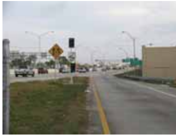
Ramp signals along I-95 will manage the rate of traffic flow entering onto the Interstate
