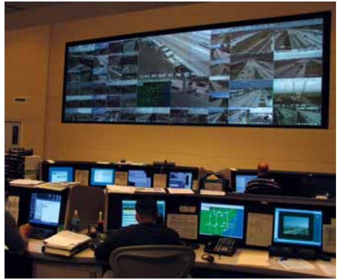
TMC Control Room
