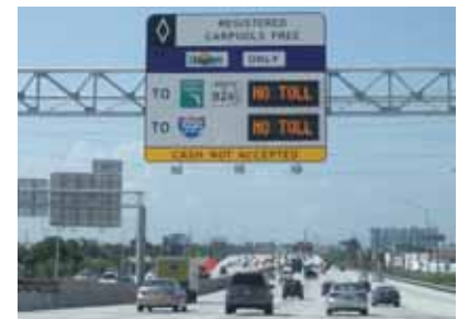
Toll rate signs will be used along the I-95 Express Lanes to advise motorists of the variable toll rate during different times of the day.
