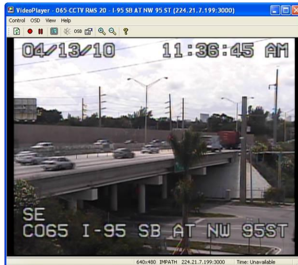
Figure 9 CCTV Preset View- Freeway
