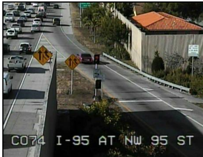
Figure 1. A Ramp Signal Implemented by FDOT
