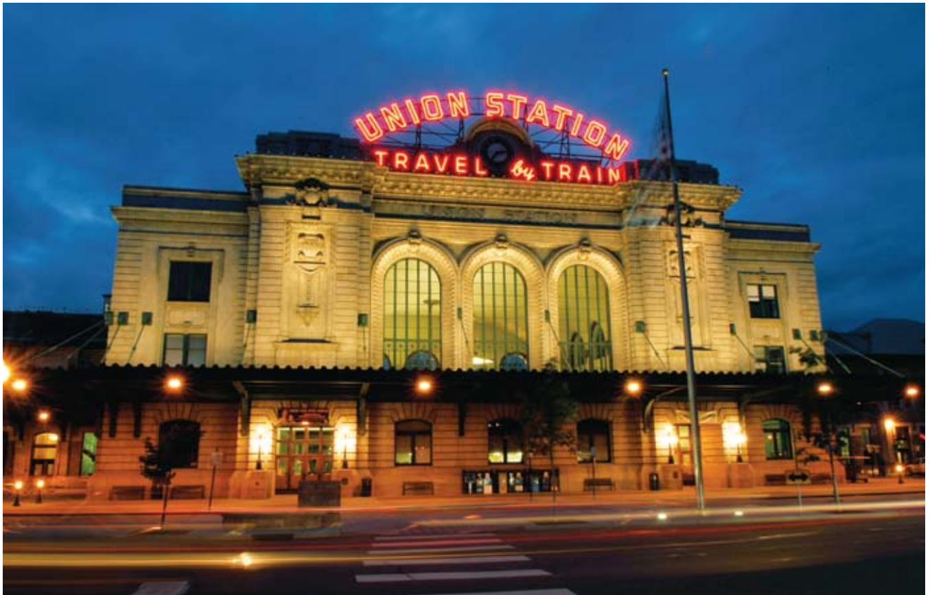
The East Corridor is almost 23 miles long, extending from a completely redeveloped Denver Union Station (pictured) to Denver International Airport. The line will have five intermediate stations, located at 38th/Blake, Colorado, Central Park, Peoria and 40th/Airport.
