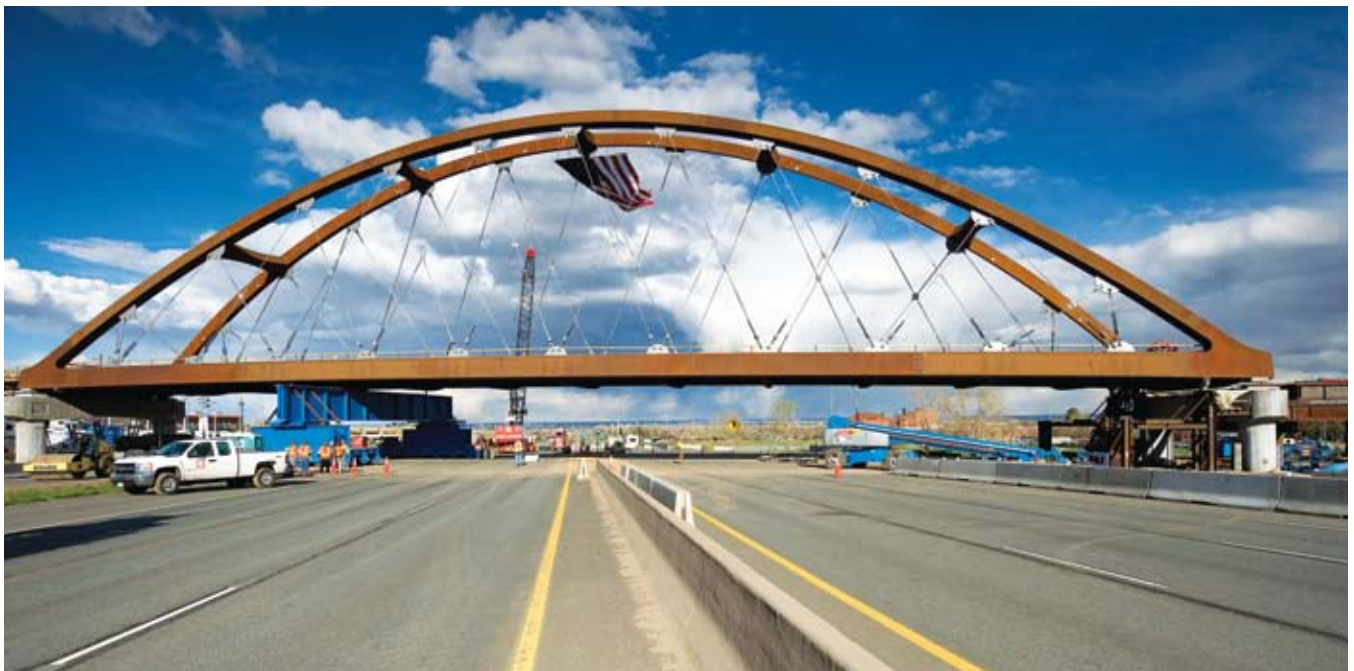
As part of constructing the West Corridor, RTD recently rolled an assembled bridge structure into place across a highway. The West Corridor is a 12.1-mile light-rail transit corridor between Denver Union Station and the Jefferson County Government Center in Golden.
