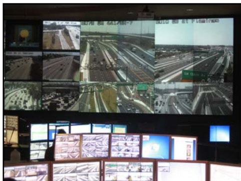
District Four transportation management center.
