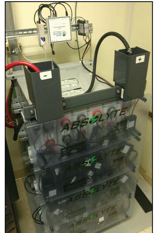
*Typical FDOT battery system with 24 individual batteries connected in series.*
