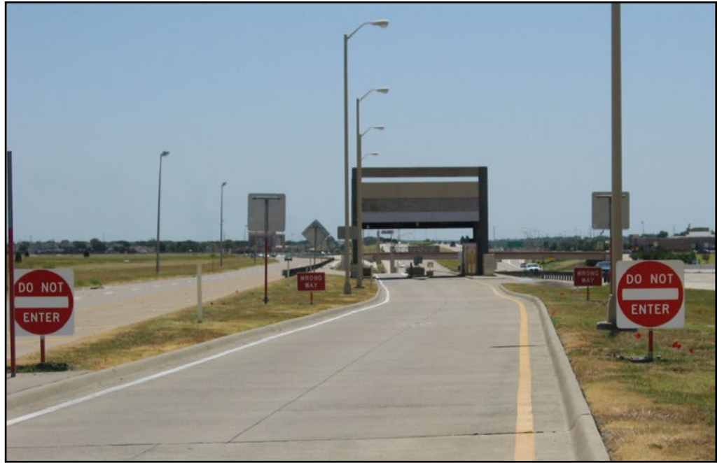
Lowered wrong-way sign.
