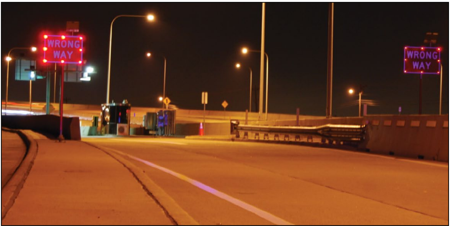
Light-emitting diode enhanced wrong-way signs.
