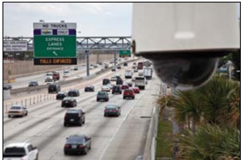
ITS technologies are critical to traffic management systems, such as 95 Express.
