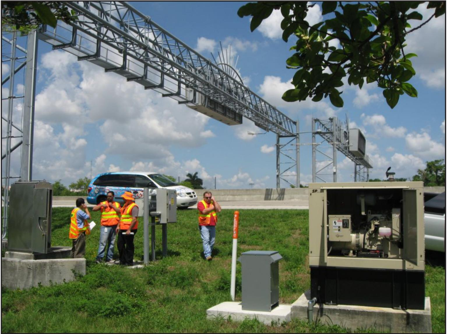
The ITS Unit quickly created and completed a list of corrective measures. The biggest lesson learned was to not be complacent and assume that a backup plan is fully functional—just because it is in place. From now on, to maintain redundant systems that are always ready for use with critical assets, the ITS Unit will perform a full system test twice a year—once before and once after hurricane season. Any time a hurricane watch is issued for the area, the test will be conducted again.
