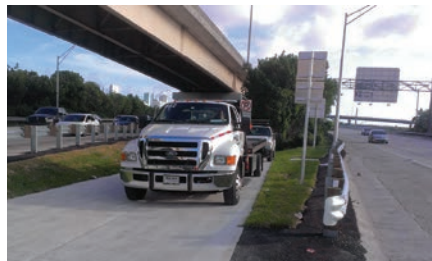
New IRV Staging Area
