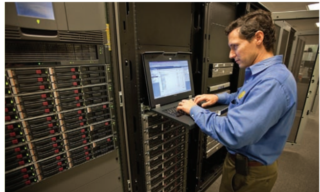
Maintenance staff at work in the SunGuide TMC server room.
