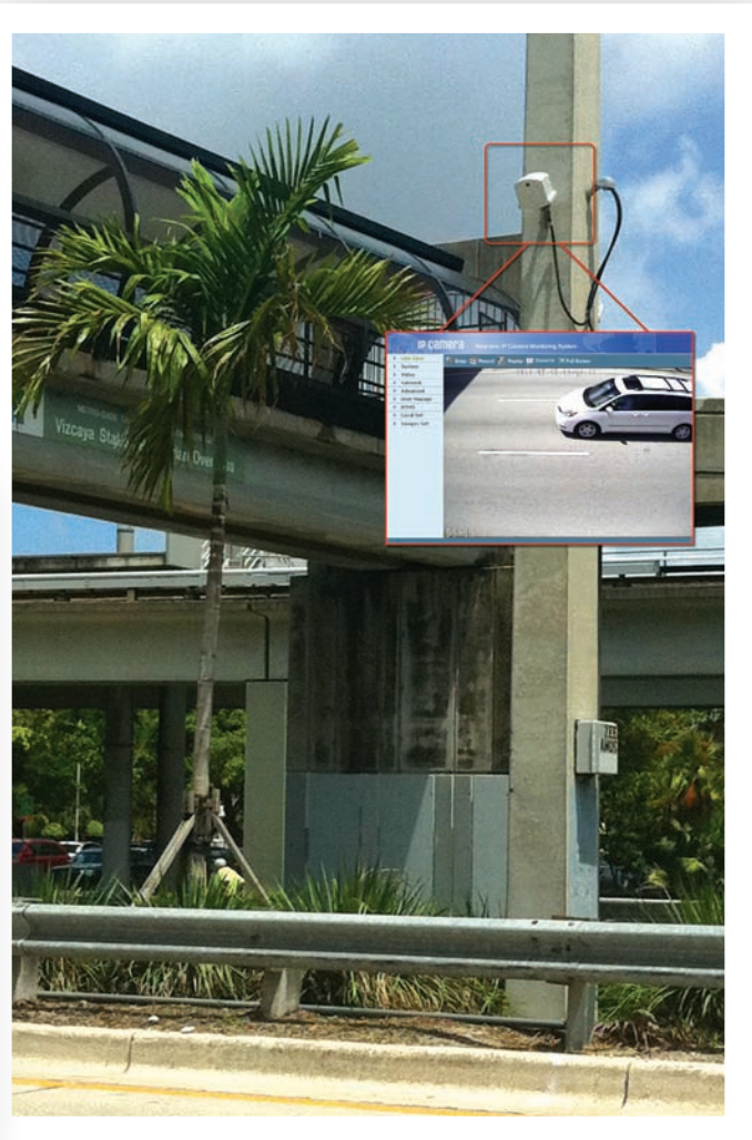
One of 31 new microwave vehicle detectors installed on I-95. The photo shows an example of what the video feed from the detector looks like.
