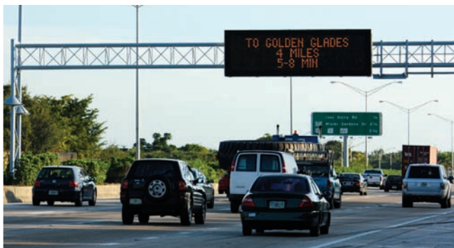
DMS displaying a travel time message on I-95 Southbound.
