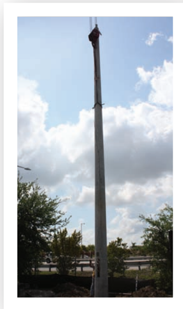
The test pole near the TMC parking lot.
