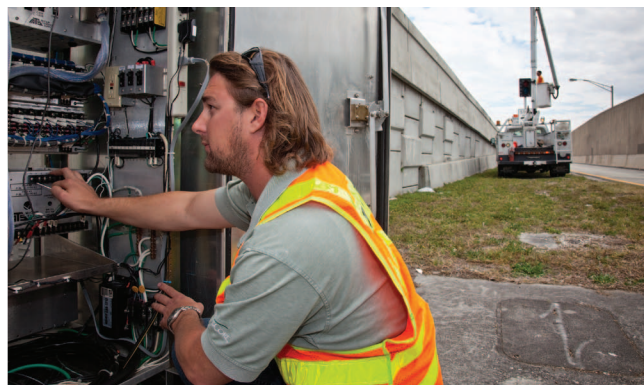
ITS Maintenance Staff works at a Ramp Signal location.
