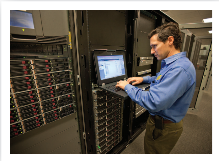
ITS Maintenance staff working in the TMC's server room.
