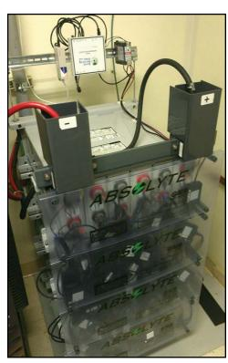
Typical FDOT battery system with 24 individual batteries connected in series.
